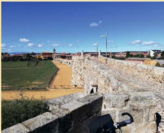
Hospital de Obrigo
